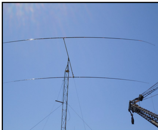
2L 20m yagi mounted on 28 ft tower at the K8O site. Antenna was fixed south-west
